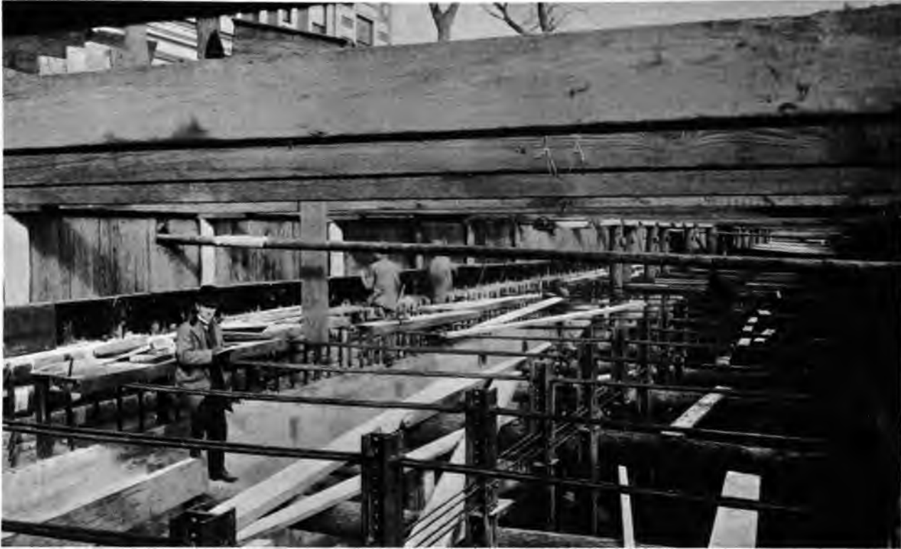
REINFORCED CONCRETE CONSTRUCTION
